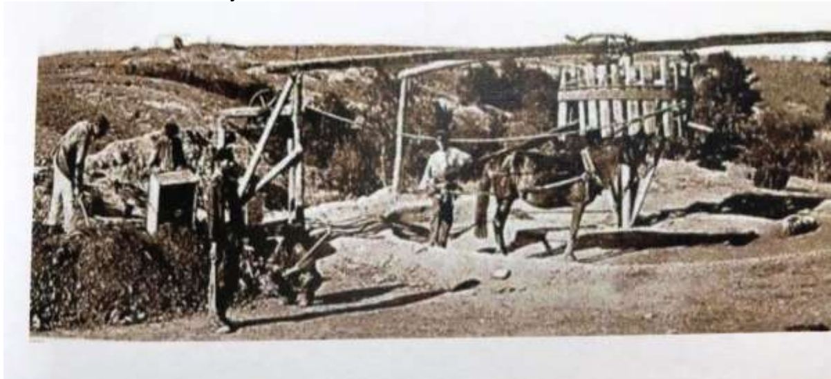
Fig. 5 – A horse-drawn drum that was used to lift iron ore [1].
