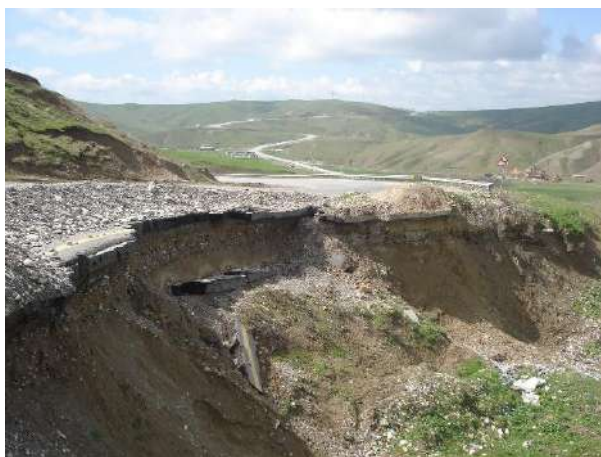
Fig. 4, 5. Landslide phenomenon at 106 km of the Baku-Gobustan-Shamakhi road (photo November 12, 2015, Tarikhazer)
