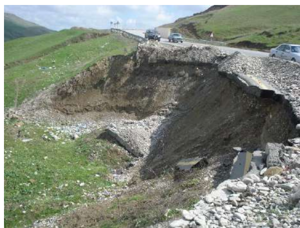
Fig. 4, 5. Landslide phenomenon at 106 km of the Baku-Gobustan-Shamakhi road (photo November 12, 2015, Tarikhazer)
