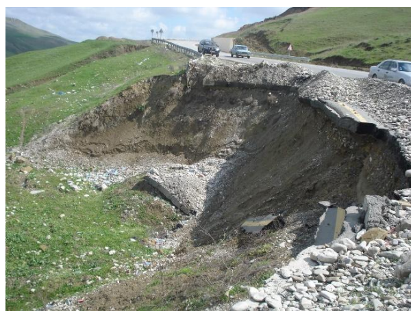
Fig. 4, 5. Landslide phenomenon at 106 km of the Baku-Gobustan-Shamakhi road (photo November 12, 2015, Tarikhazer)
