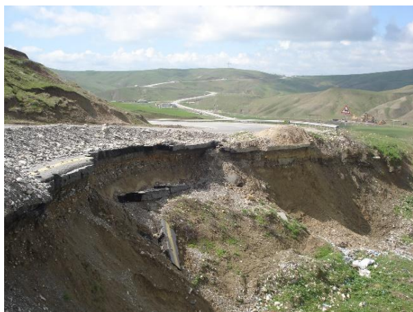
Fig. 4, 5. Landslide phenomenon at 106 km of the Baku-Gobustan-Shamakhi road (photo November 12, 2015, Tarikhazer)
